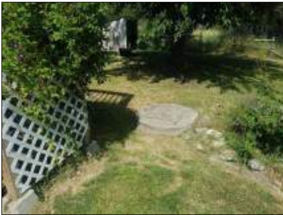
Photo 11. Septic tank located behind house.
